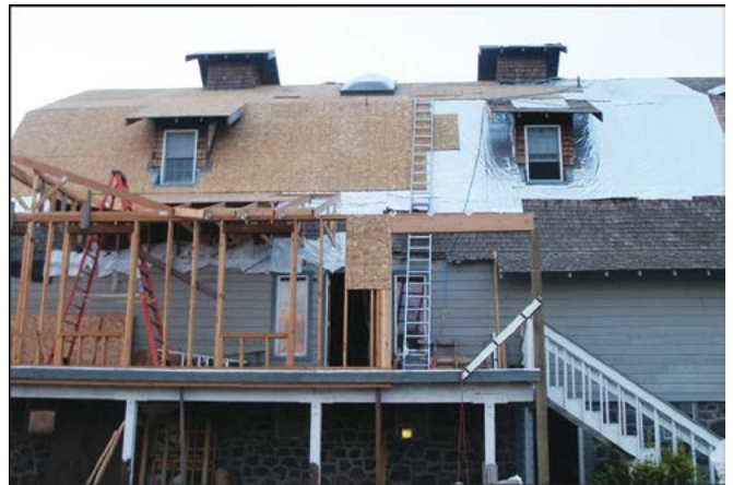
The product also is extremely valuable for energy savings in existing structures. In this photo it is seen that the reflective is being installed on top of old roofing before new roofing is applied. The result is very high savings in both heating and cooling costs for the home.
