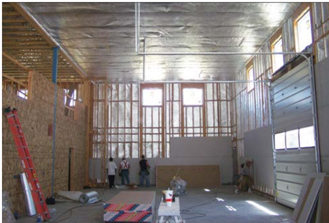
The bigger the building the bigger the savings when it comes to use of reflective aluminum foil which keeps out over 97% of the heat from the sun. In this commercial building the reflective foil is applied under sheathing and prior to the installation of drywall for maximum savings.
