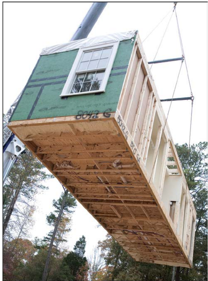
Setting a modular section by crane. New World Home offers a move-in schedule of approximately 100 days in most locations. The homes are produced on-demand eliminating the problems associated with an unsold inventory.
